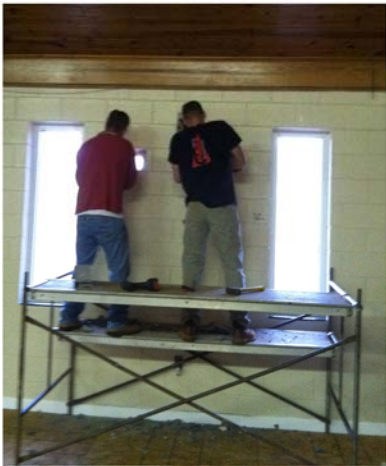
Removing blocks from inside to facilitate new door
