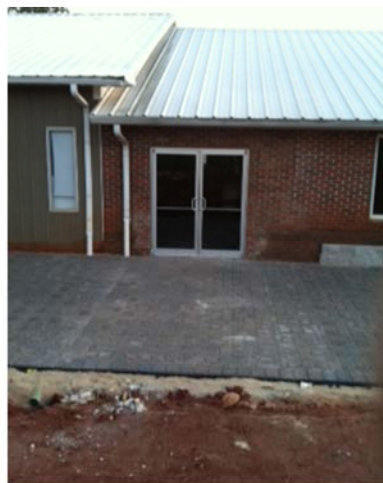
Temporary glass doors--permanent doors on order.
