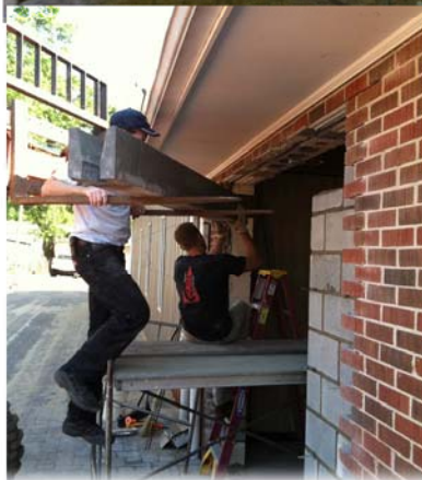
Installing bond beam above where the new door would be
